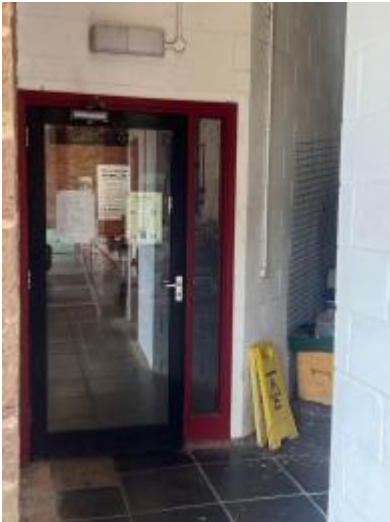
entrance to gallery 5 from ramp on level 1
