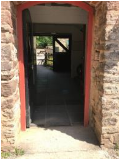
access through mill building towards cottage
