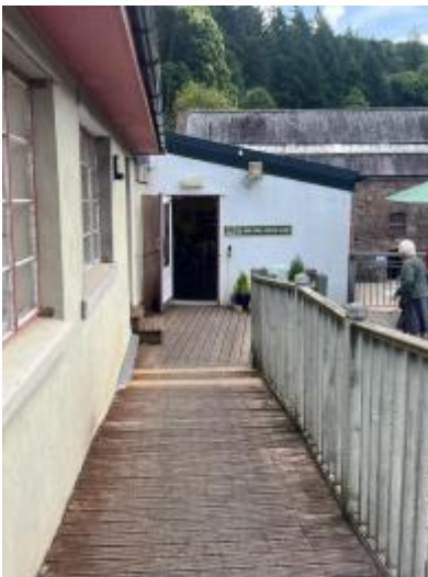
decking ramp to coffee shop
